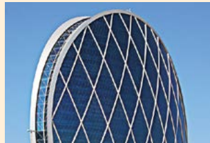
Al Dar Headquarters, Abu Dhabi
